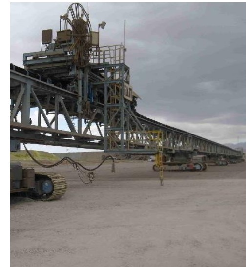
Spence Interim Fatigue Strengthening
