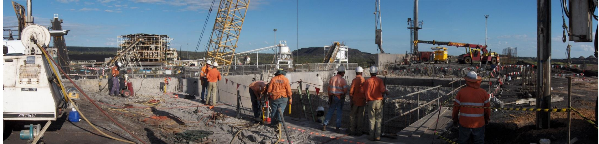
Peak Downs ROM Upgrade for Cat 797 Dump Trucks
