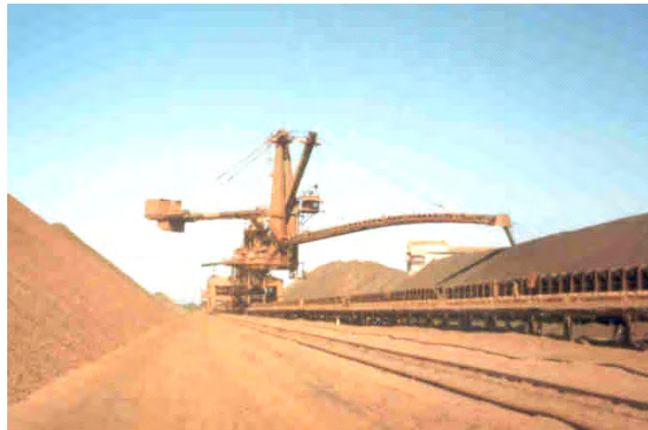
Figure 6: Stacker with luffing winch
