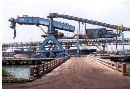
Figure 3: Portal slewing and shuttling shiploader
