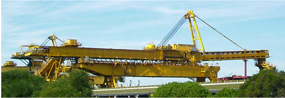
Figure 1: Long travelling bridge type shiploader
