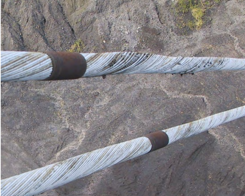
Figure 16: Damaged stays
