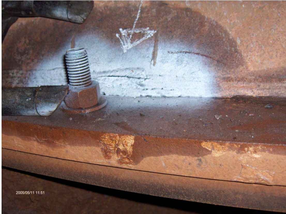
Figure 14: Fatigue cracking
