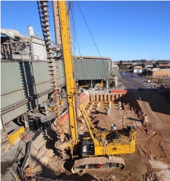
Figure 5 – CFA Piling Rig
