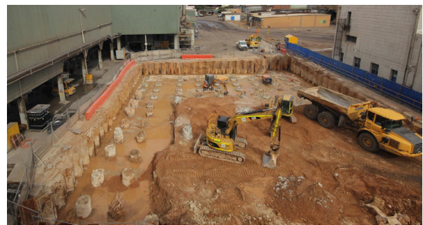
Figure 6 – Post Piling Excavation
