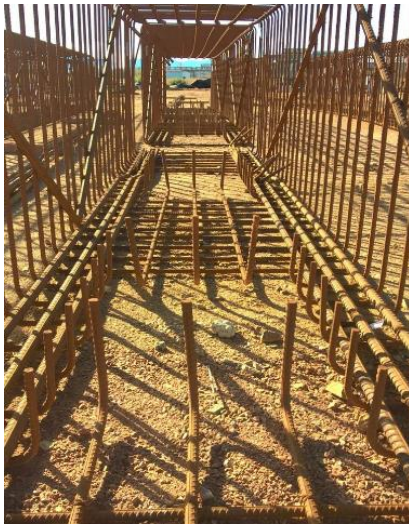
Figure 7 – Reinforcement Cage
