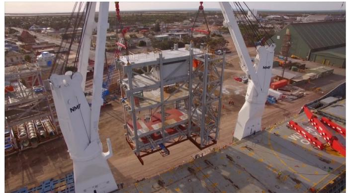
**Figure 7: Module Lifting – Ship to Shore**
