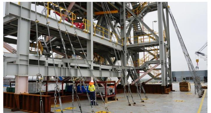
**Figure 5: Module Lashed to Ship Deck**
