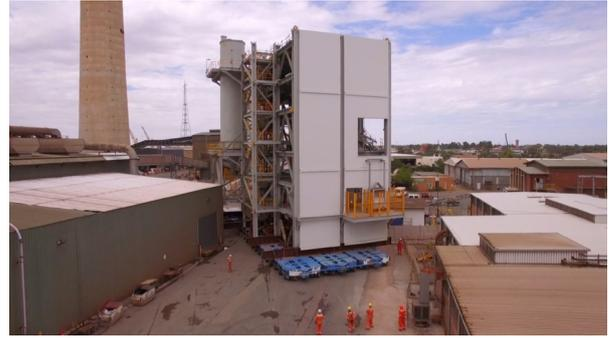
**Figure 3: Moving Modules on Site**
