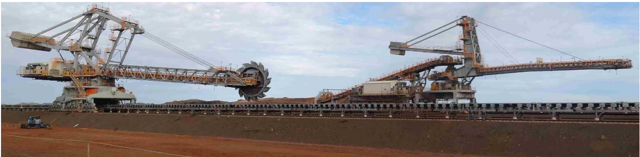
Figure 1: Reclaimer and Stacker for Iron Ore
