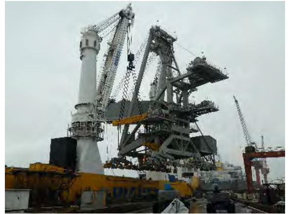
Shiploader being lifted onto heavy lift ship
