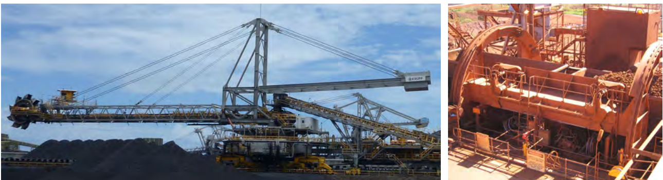
Stacker Reclaimer (Left), Car Dumper (Right)
