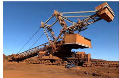
Reclaimer 1 Rio Tinto Iron Ore Parker Point
