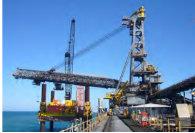
Shiploader SL1 BHP – Hay Point Coal Terminal
