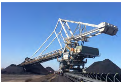
Reclaimer RC821 BMA Caval Ridge Mine
