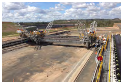
Bridge Reclaimer BMA Caval Ridge Mine
