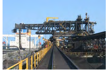
Shiploader SL2 BHP – Hay Point Coal Terminal
