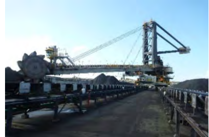
Stacker Reclaimer SR5 Darlymple Bay Coal Terminal
