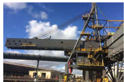
Berth 8 Shiploader Port of Townsville
