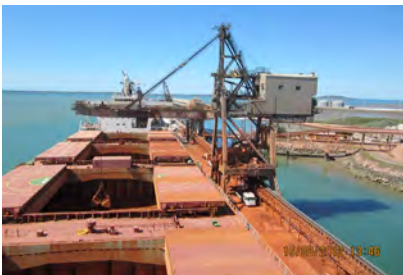
Ship Unloader 2 Queensland Alumina Limited
