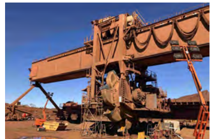
Bridge Reclaimer Rio Tinto Iron Ore Paraburdoo
