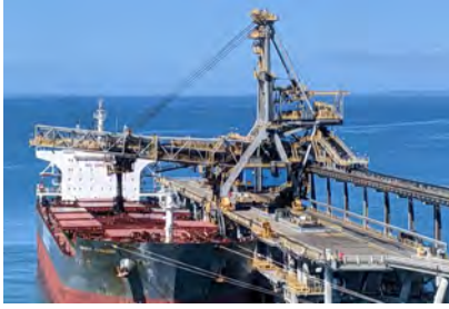
Shiploader 3 Hay Point Coal Terminal
