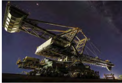
12,500 TPH Reclaimer Rio Tinto Alcan – Amrun Project
