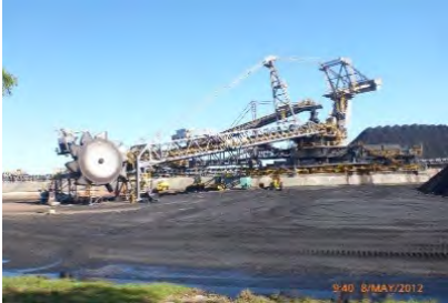
Stacker Reclaimer SR0 BMA Hay Point Coal Terminal
