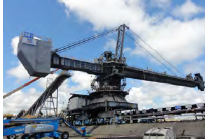
Stacker Reclaimer SR1 BMA – Hay Point Coal Terminal
