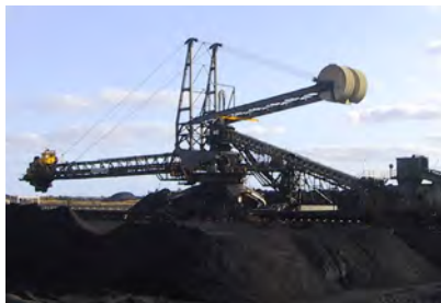
Stacker Reclaimer SR1 Darlymple Bay Coal Terminal
