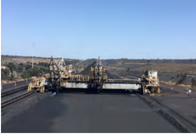
Raw Coal Reclaimer BMA – Goonyella Riverside Mine
