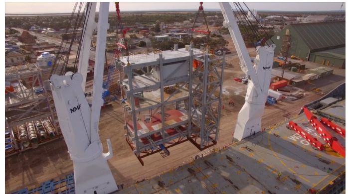
Figure 7: Module Lifting – Ship to Shore
