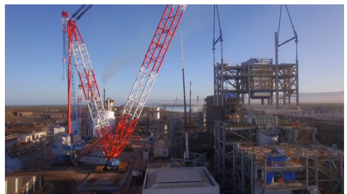
Figure 8: Module Lifting – Installing in Building
