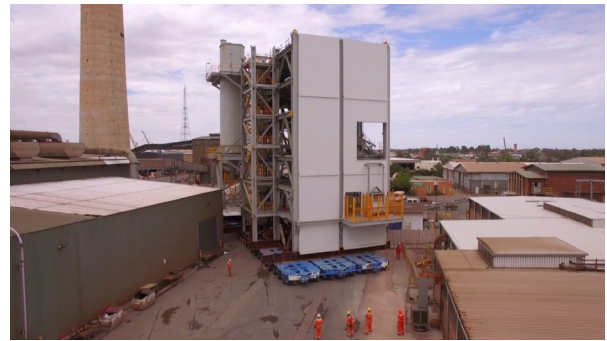
Figure 3: Moving Modules on Site
