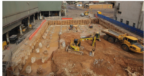
Figure 6 – Post Piling Excavation
