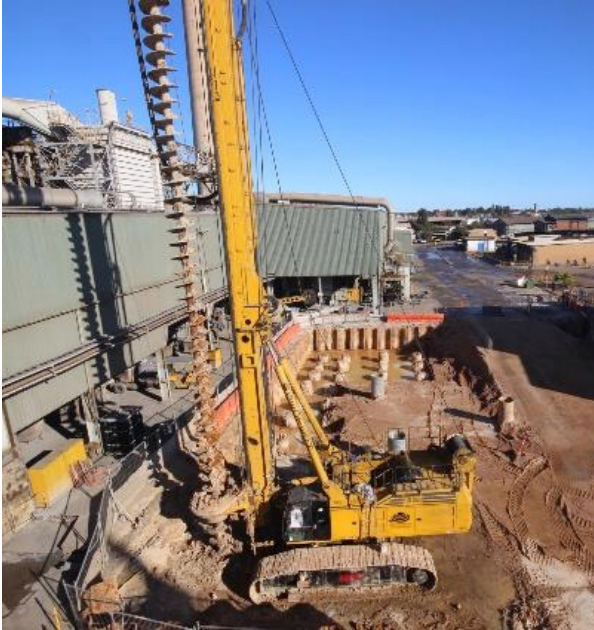
Figure 5 – CFA Piling Rig
