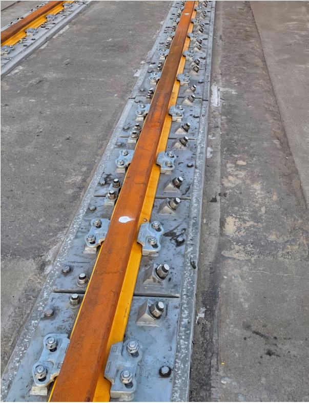
Figure 4. Completed sole plate installation after grouting and rail installation.
