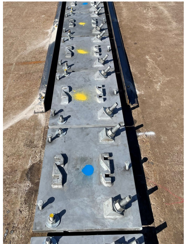
Figure 1. Rail sole plates during installation.
