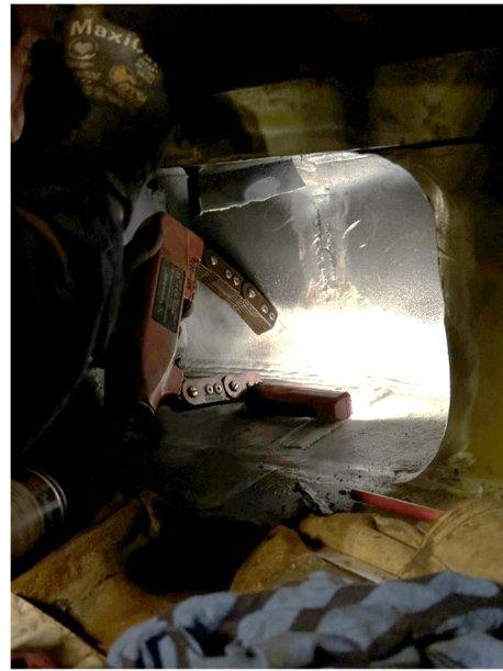
Figure 4. Circular box girder modifications to conduct crack repairs on a reclaimer at iron ore mine site in WA.
