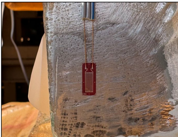
Figure 1 – Strain gauge installed on the long travel structure of a bucket wheel reclaimer.
