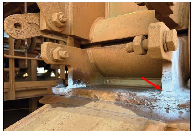
Figure 6 – Cracking of long travel bogie pillow block.
