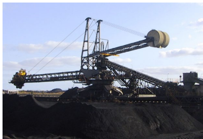
Stacker Reclaimer SR1 Darlymple Bay Coal Terminal
