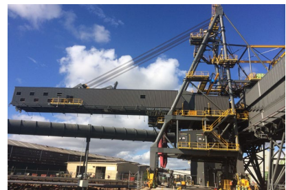
Berth 8 Shiploader Port of Townsville
