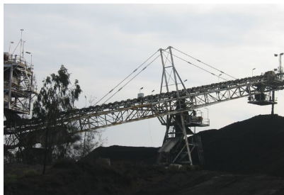
Radial Stacker Peak Downs Mine
