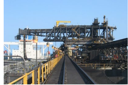
Shiploader SL2 BHP – Hay Point Coal Terminal
